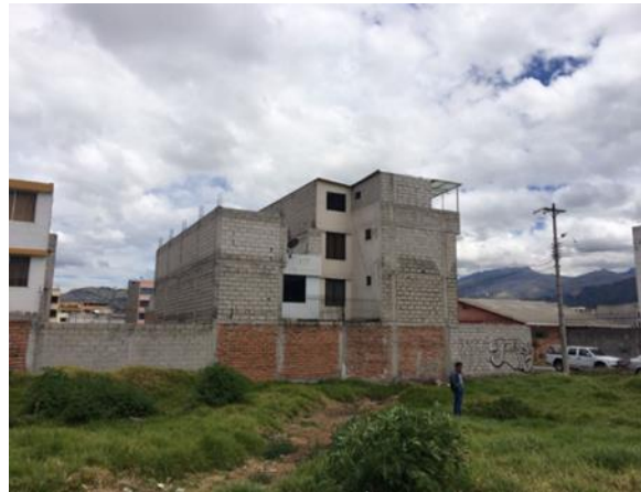
Figure 3: Existing conditions of site before development.
