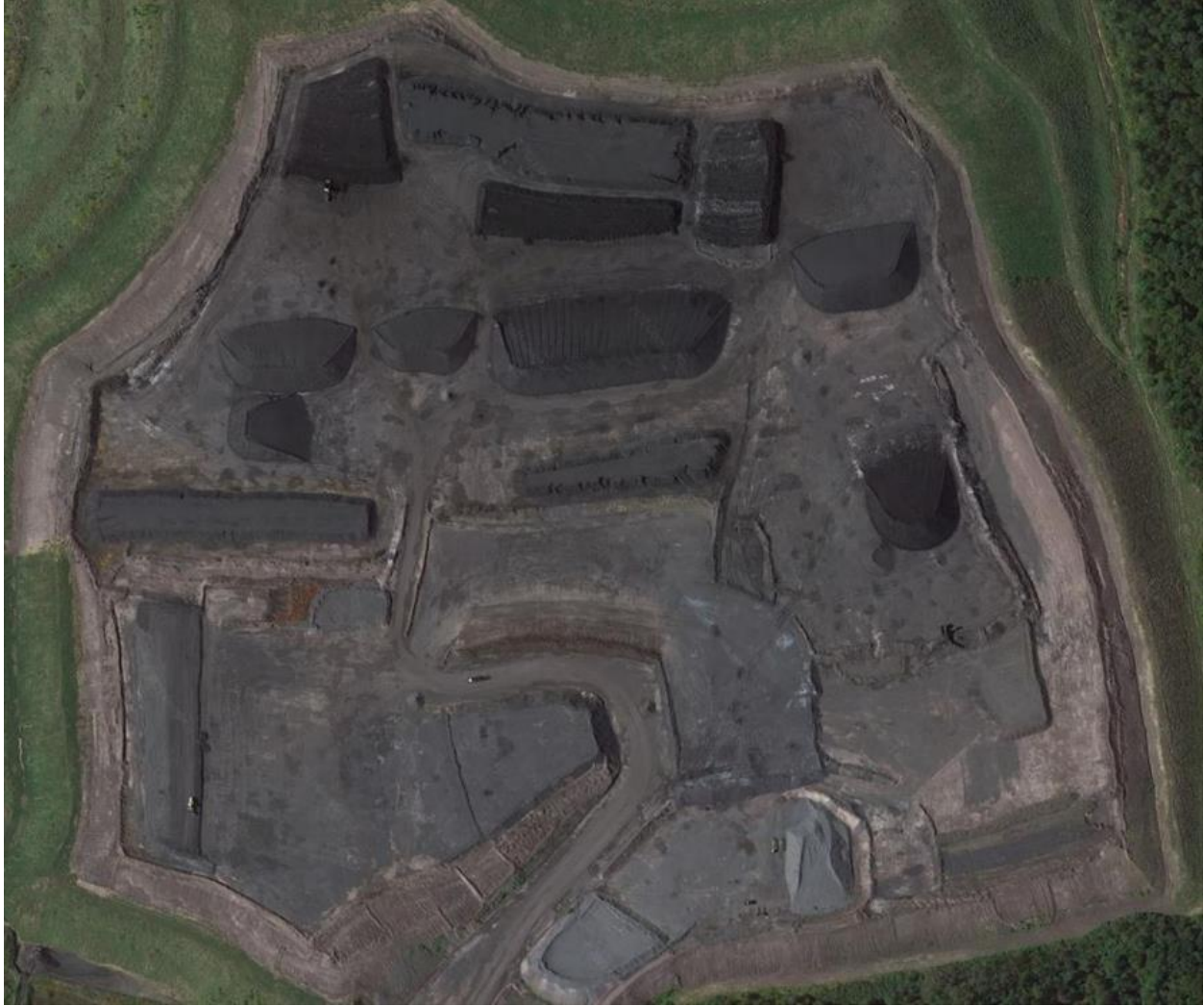
Figure 4: Google Earth picture of Cambria Slope No. 33
