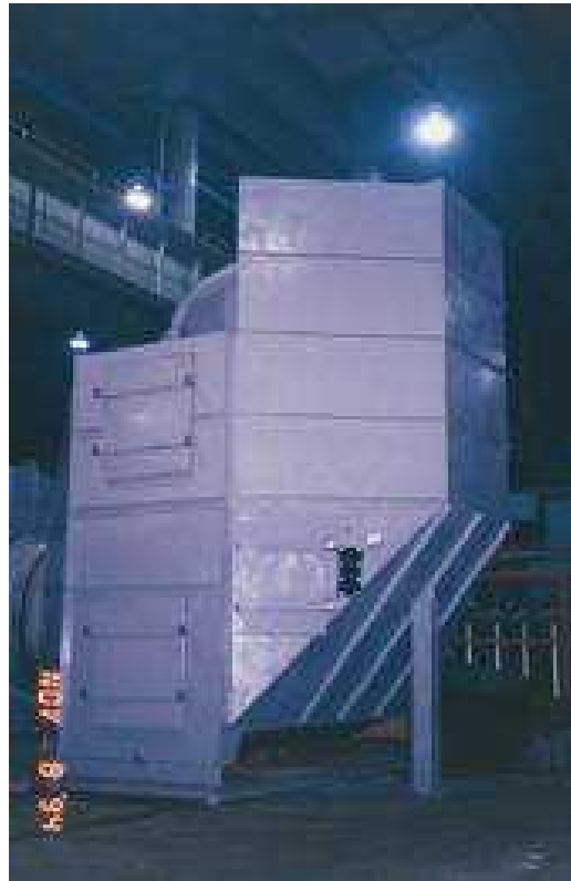
Figure 33: Oil mist eliminator
