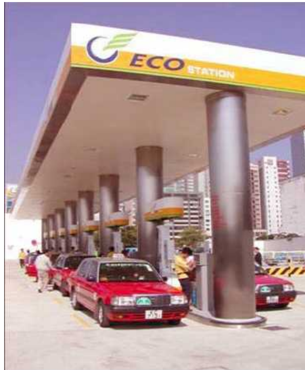
Figure 45: LPG Filling Station in Hong Kong
