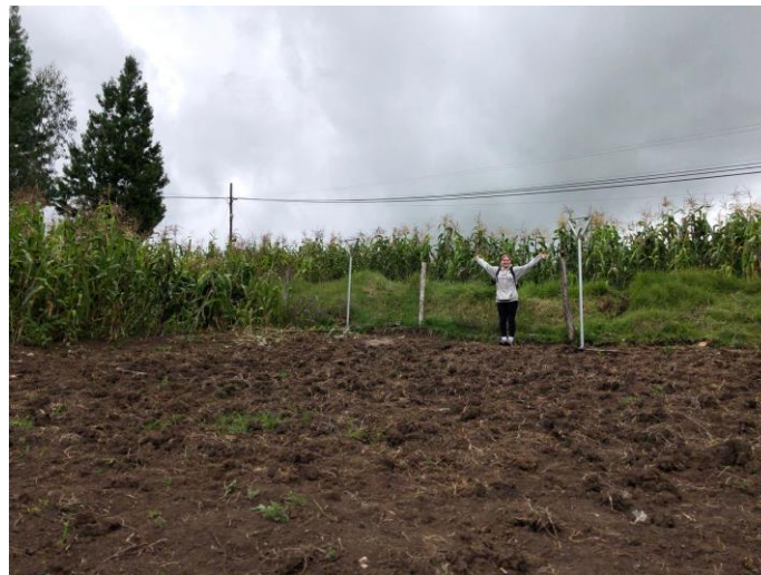
Figure 6: Victoria del Portete Greenhouse Site under Construction, Taken by Emiliano
