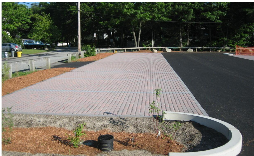
Figure 4.2: Permeable pavers, porous asphalt, and bioretention cells at the Silver Lake beach parking lot, Wilmington MA (Demonstration 3, n.d.)
