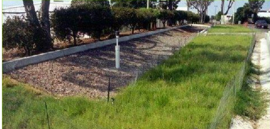
Figure 4.1: Grass filter strip is being used as pretreatment for parking lot runoff directed to an infiltration basin. Note concrete level spreader (at right) to facilitate sheet flow across the filter strip (Fact Sheet, n.d.)
