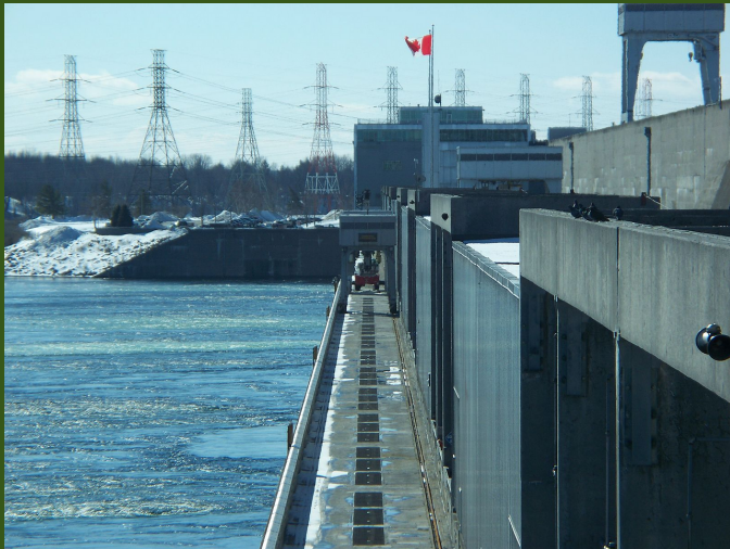
Figure 9: OPG's RH Saunders generating station on the St. Lawrence River (ceedub13, 1998)
