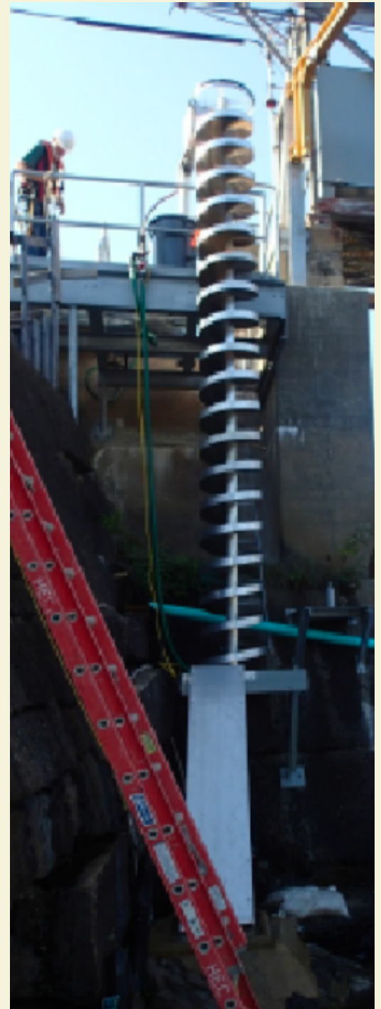
Figure 5: Helical eel ramp (Anonymous conservationist, personal communication, February 4, 2021. Reprinted with permission.)
