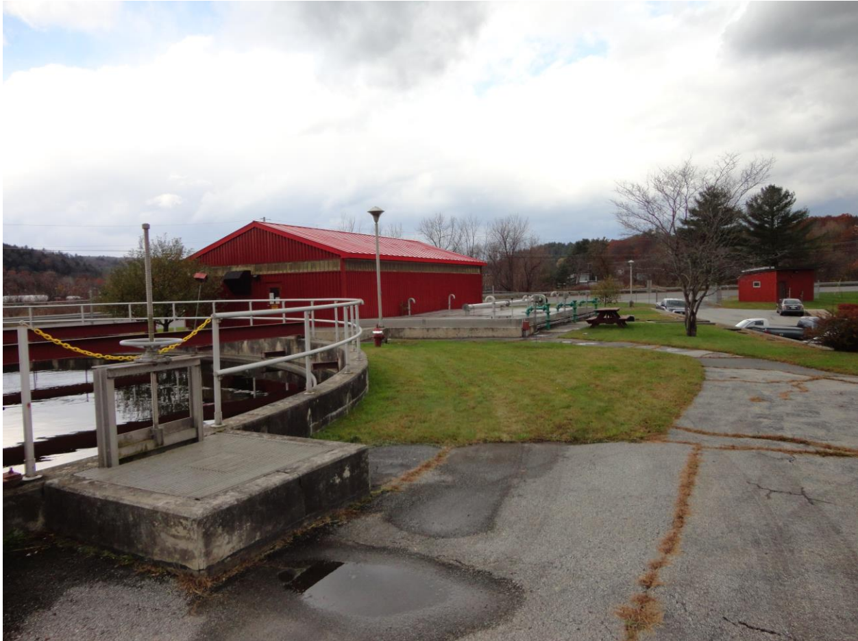
Figure 18: Secondary clarifier in the foreground with UV disinfection building and existing sludge holding tanks in background at the Montpelier WWTF
