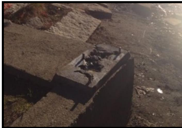
Figure 63: Pedestal erosion
