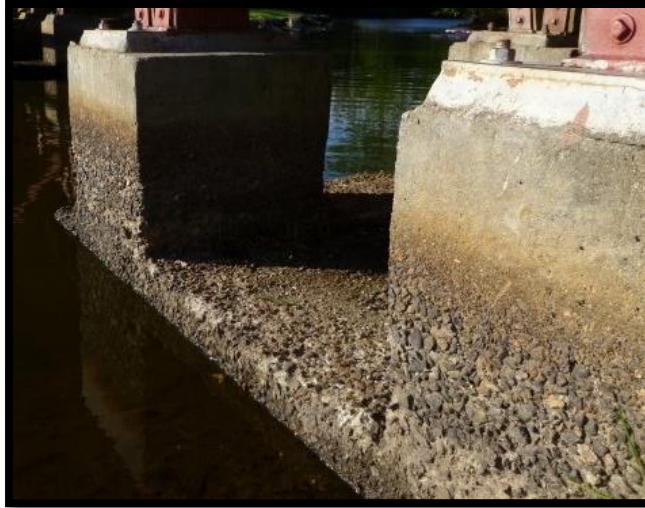
Figure 62: Foundation erosion.
