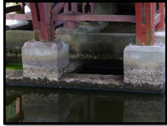
Figure 65: Image of current bridge footings - wide view of multiple piers.
