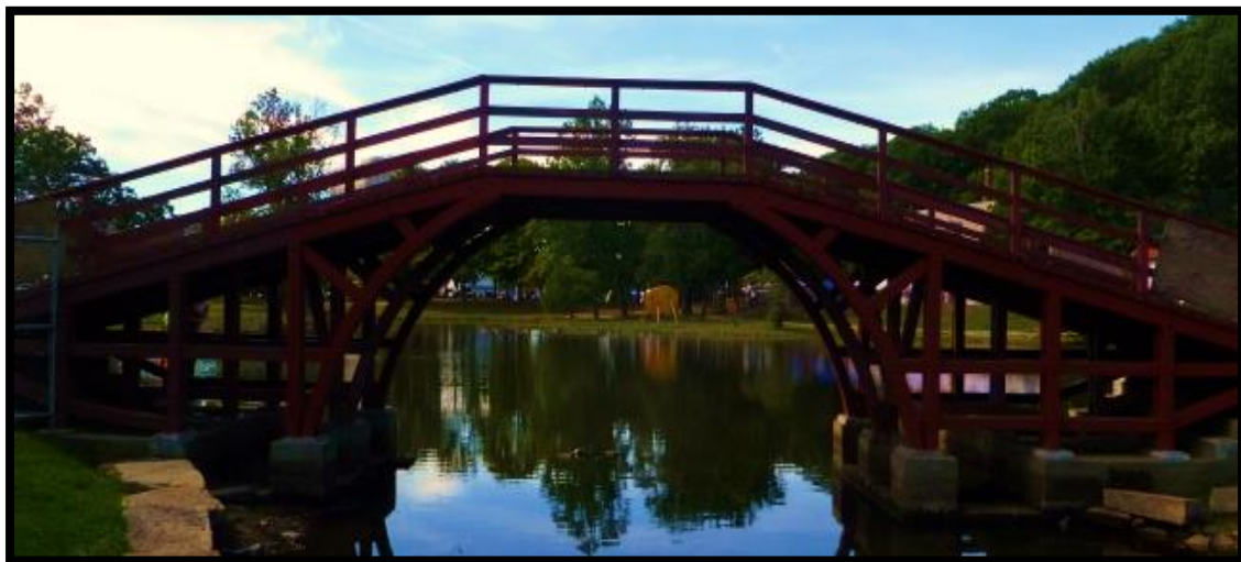
Figure 15: Image of Elm Park Red Wooden Bridge (September 2013).
