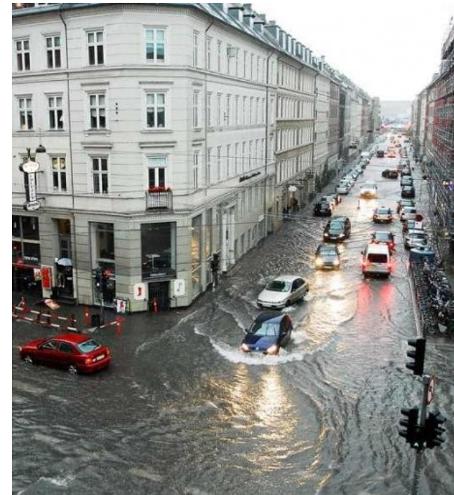
Figure 2: Cloudburst flooding on a Copenhagen street, 2011 5
