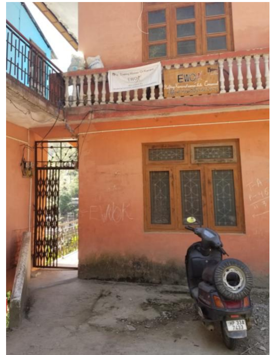
Figure 2. EWOK offices (photo credit: Savrin, 2019)
