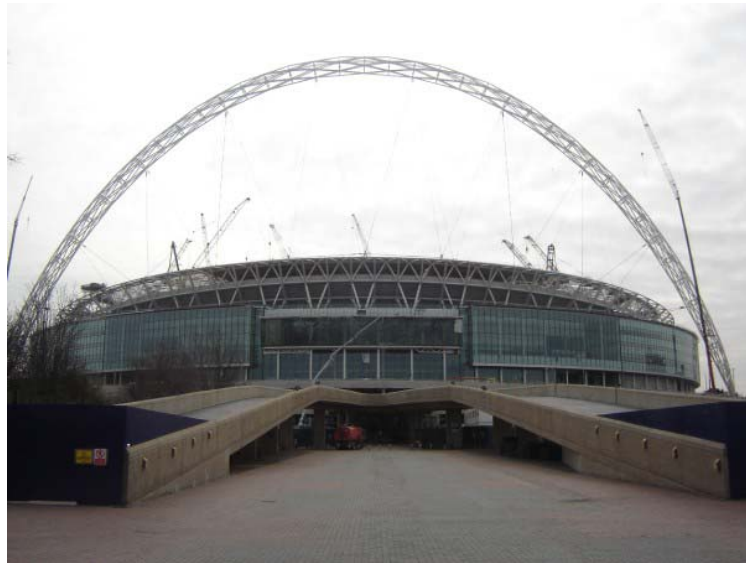
Figure 1: Wembley Stadium March 2006
