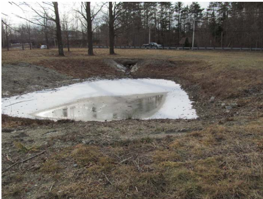
Figure 45: Gate 25 Basin Forebay
