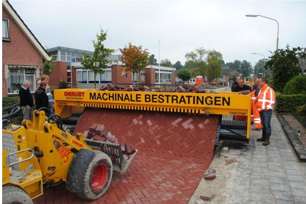
Figure 12 – Bricklaying Robot: Roads
