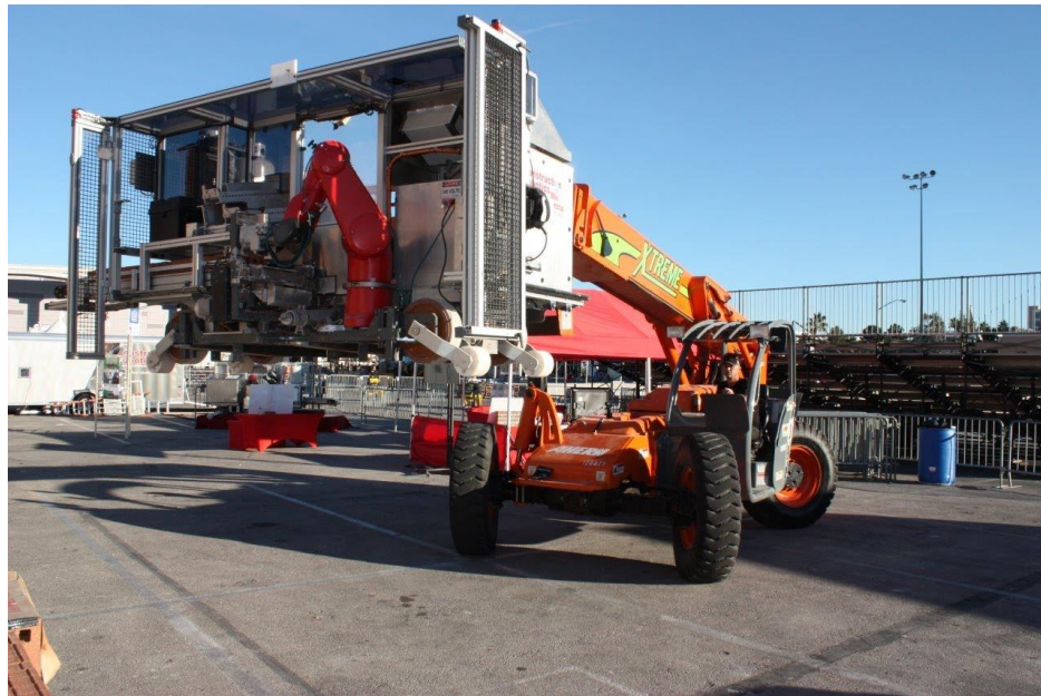
Figure 11 – Bricklaying Robot: Walls
