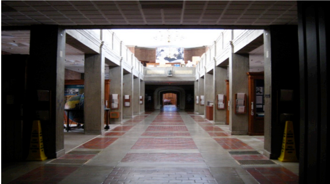
Figure 2: A Change in Floor Texture Indicates a Path to the Left and Right.
