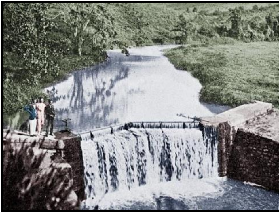
Figure 21. The weir of the Antiguo Acueducto from around the year 1918. This image is from the Trust's archives.
