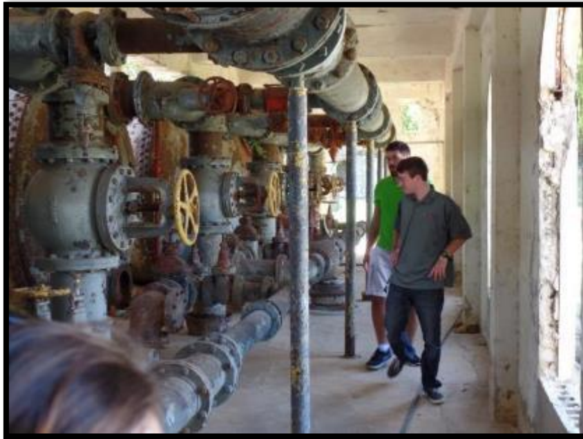
Figure 9. Site of the Antiguo Acueducto. (a) Water filter tank that belongs to the site of the Antiguo Acueducto and was acquired later by Trust after being taken from the site. (b) Current condition of the mechanical water filtration system.
