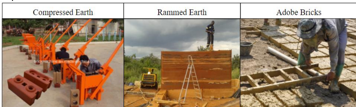
Figure 5: From left to right: compressed earth machine and bricks (Henry Industrial Co., Ltd., 2015), rammed earth method (the Akaa project, 2015), and adobe method with formwork (CLC, 2011).
