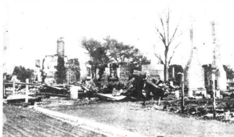
DERRINALLUM'S MAIN STREET also looks the same as it did immediately after the January holocaust. A recent three-day tour of this part of the Western District revealed the fact that the foundations of not more than 20 of every 100 homes destroyed have been laid.
