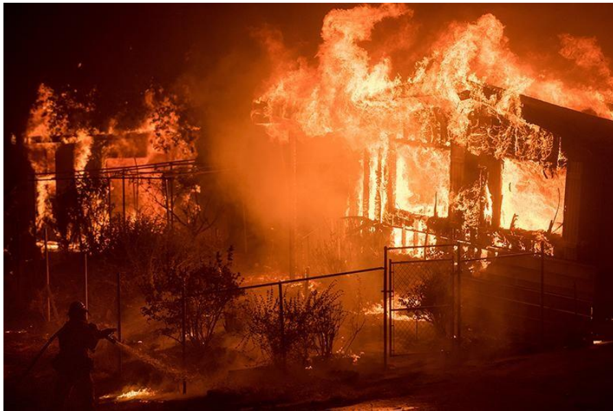
SafetylineJalousie. (2018, September 13). Bushfire Rated Houses Burn Down Causing Some Experts To Question Building Regulations. Retrieved from https://safetylinejalousie.com.au/bushfire-rated-houses-burn-down-causing-some-experts-to-question-building-regulations/
