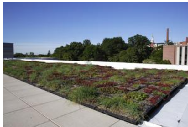
Figure 10 Green Roof over East Hall (East Hall Sustainable Features, 2009)
