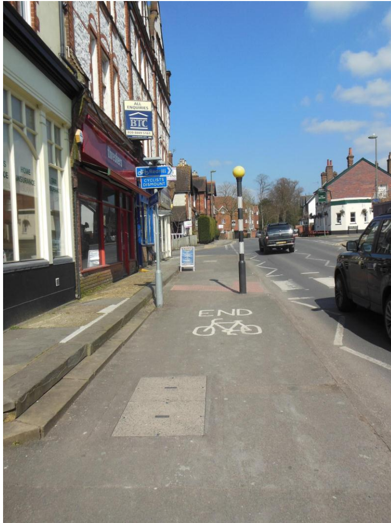
Figure 19: Abrupt ending of the cycle lane on Croydon Road
