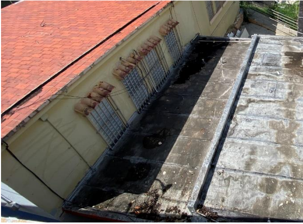
Roof #4 Area: 288 sq.ft. Obstructions: Heavily shaded
