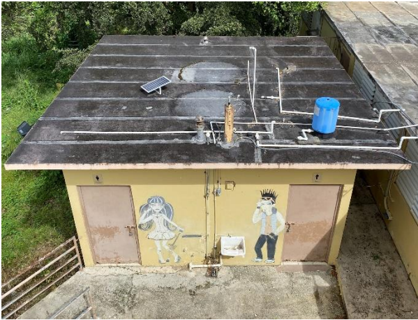
Roof #6 Area: 463 sq.ft. Obstructions: Column, pipes
