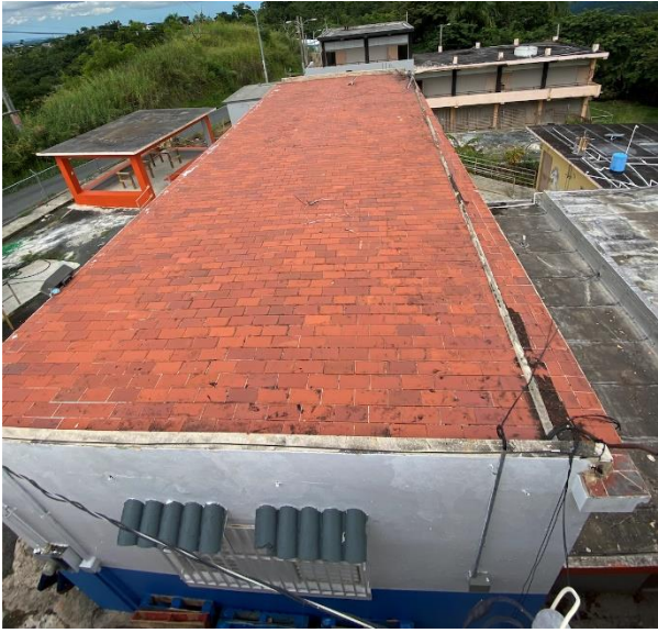
Roof #3 Area: 1283 sq.ft. Obstructions: None
