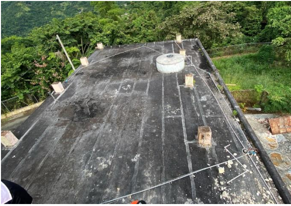
Roof #7 Area: 1652 sq.ft. Obstructions: Columns, old water tank
