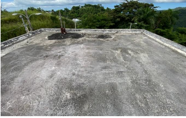
Roof #8 Area: 821 sq.ft. Obstructions: None
