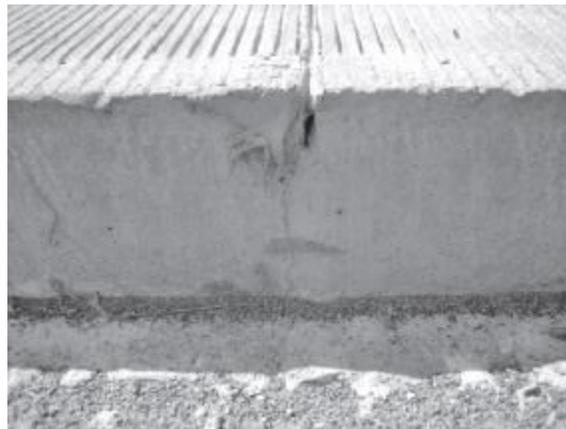
Figure 8: Precut joint in concrete Slab with polymer filling (El-Korchi & Mallick, 2013)
