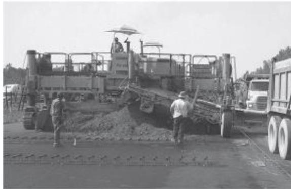
Figure 5: Pouring Concrete using a concrete paver to form the pavement (El-Korchi & Mallick, 2013)
