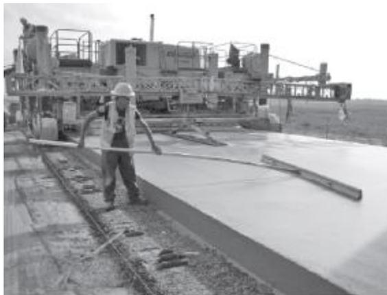
Figure 6: Finishing the pavement slab surface using a bullfloat (El-Korchi & Mallick, 2013)
