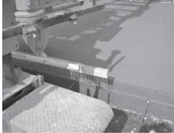
Figure 7: Creating Grooves in the Pavement using a steel comb apparatus (El-Korchi & Mallick, 2013)
