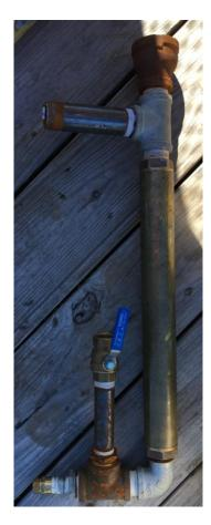
Figure 35: Fill Point Assembly
