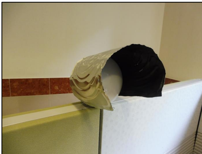
Figure 37: Aluminum Shield added to a Dome Light
