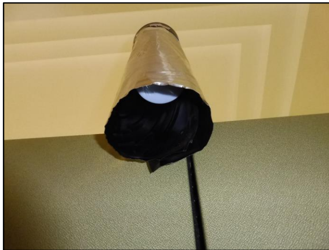
Figure 35: Aluminum Shield added to a Pickle Jar Light
