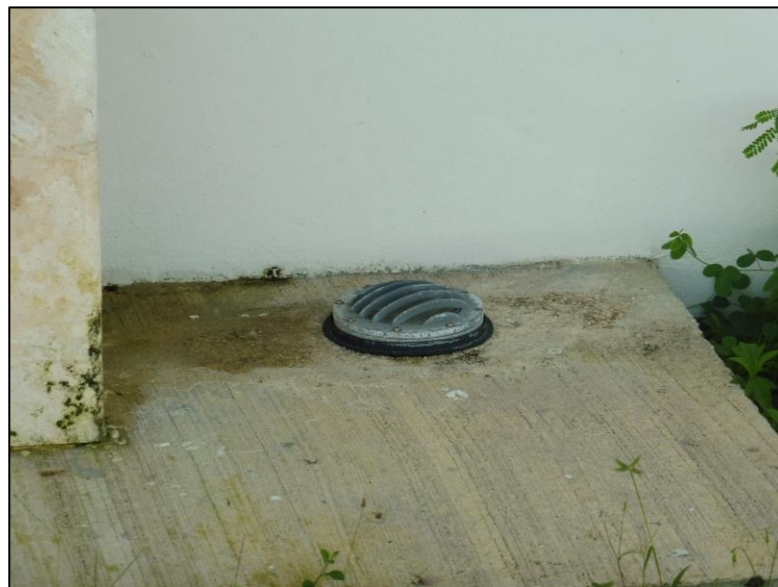
Figure 44: Dome Light set in the Ground
