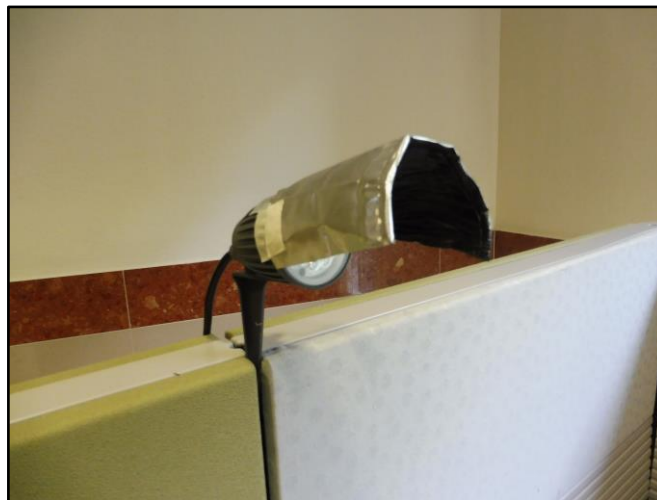
Figure 31: Small Aluminum Shield added to the Circular Spotlight
