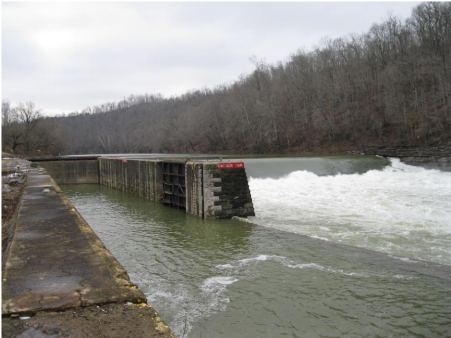
Figure 1: Kentucky River Lock and Dam No. 8
