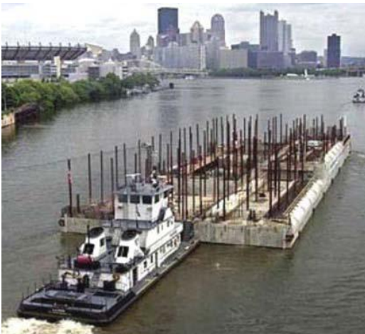
Figure 5: Floating segment for Braddock Dam
