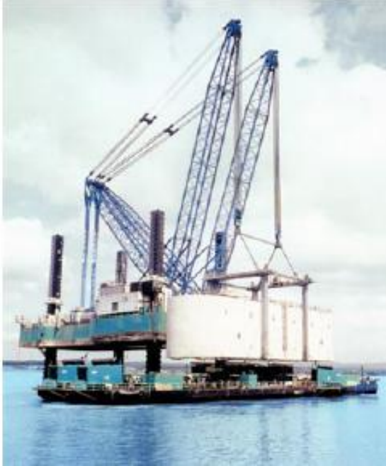
Figure 6: Crane Barge (Ben C. Gerwick Inc., 2000)
