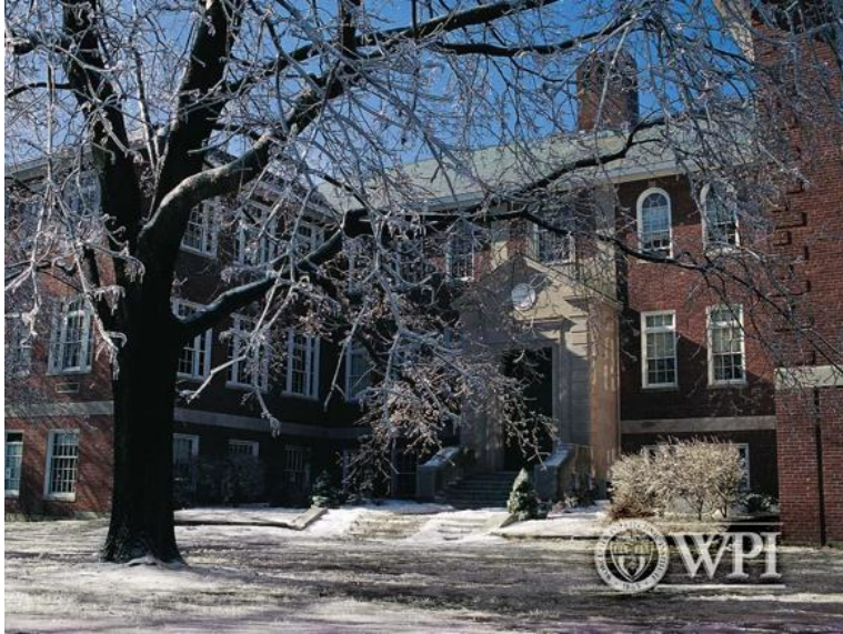
Photograph of Kaven Hall, for reference with above proposed administration building. 32
