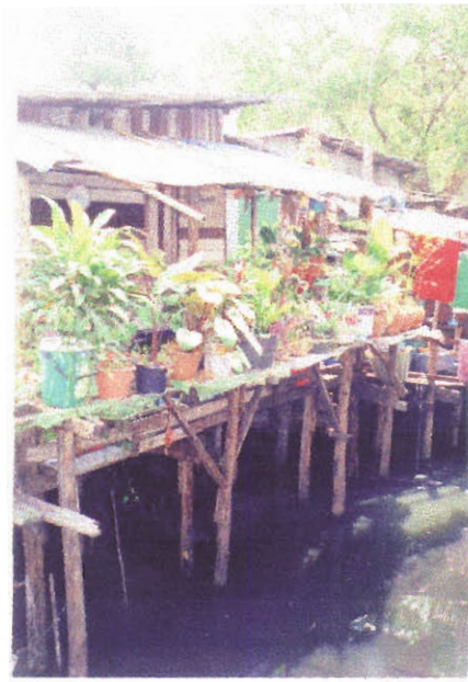
Figure 3: Houses Above a Canal
