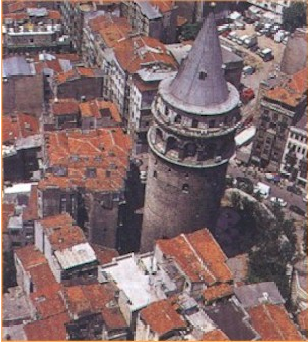
Figure 3-9 Many Unplanned Buildings Crowding Historic Galata Tower in Beyoglu, Istanbul
