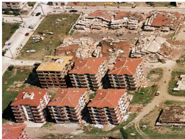
Figure 3-14 Structurally Unsound Buildings after Kocaeli Earthquake in 1999
