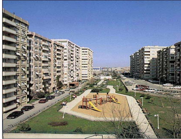
Figure 3-22 High-rise Construction with Open Space
