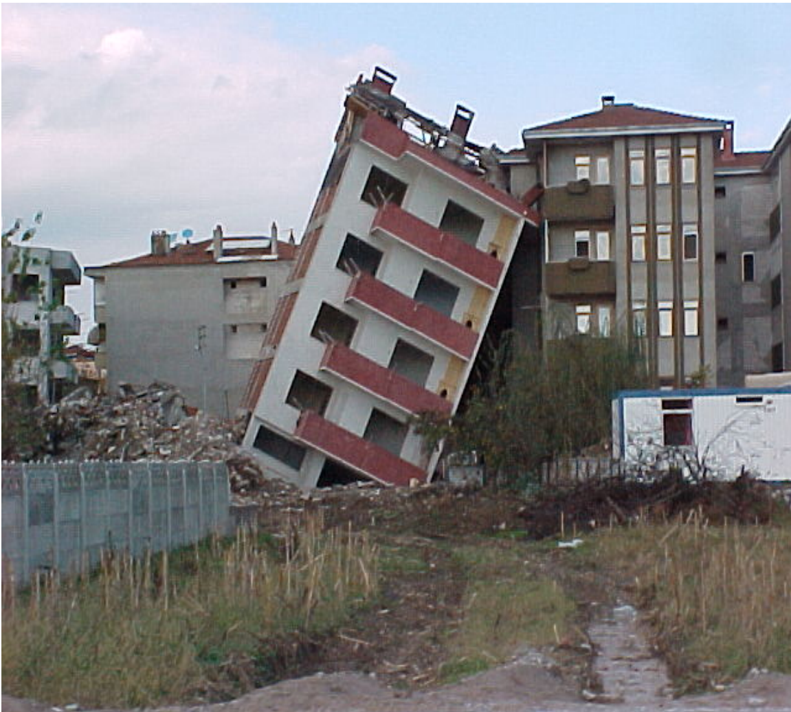
Figure 3-4 Newly Constructed Building Tilted due to an Earthquake
