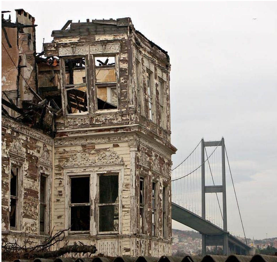
Figure 3-10 A Typical Historic Villa ruined due to Lack of Restorations
