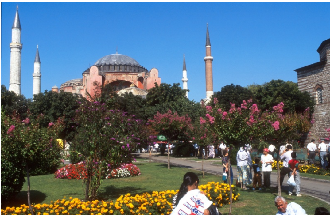
Figure 3-38 Elimination of unauthorized and undesirable buildings around historical sites will reintegrate the history with nature
