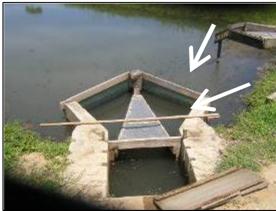
Figure 7-5 Double filtration system with multiple nets located at an inlet gate.
