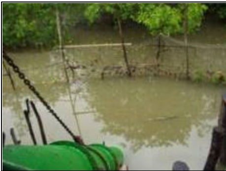
Figure 1-2 Example of netting used to keep debris out of the inlet.
