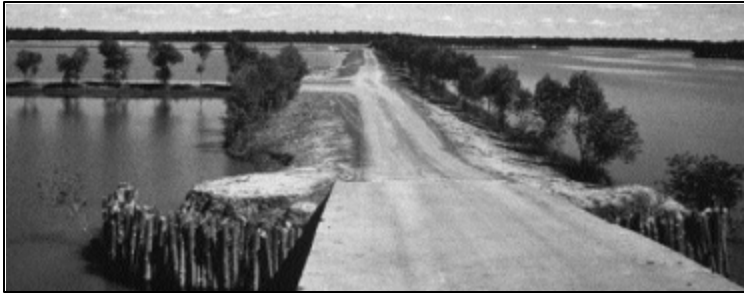
Figure 7-1 An example of mangroves used to prevent erosion along roads and retaining walls 14 .
