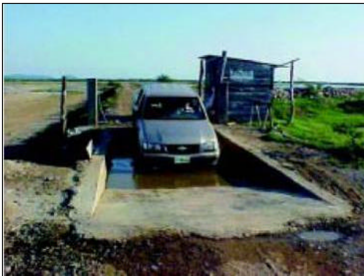
Figure 7-2 An example of a vehicle washing station on a shrimp farm 15 .
