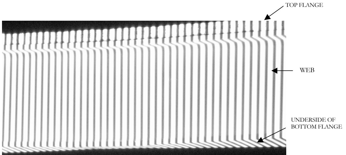
Figure 17. Damaged Aluminum I-beam with fringe pattern projection demonstrating distortion of fringes.
