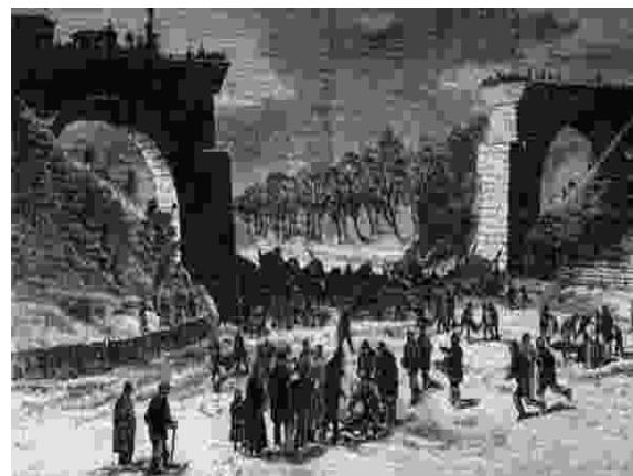
Figure 5. Drawing depicting the night of the bridge collapse. Reprinted from the Ashtabula Railway Historical Foundation web page.
