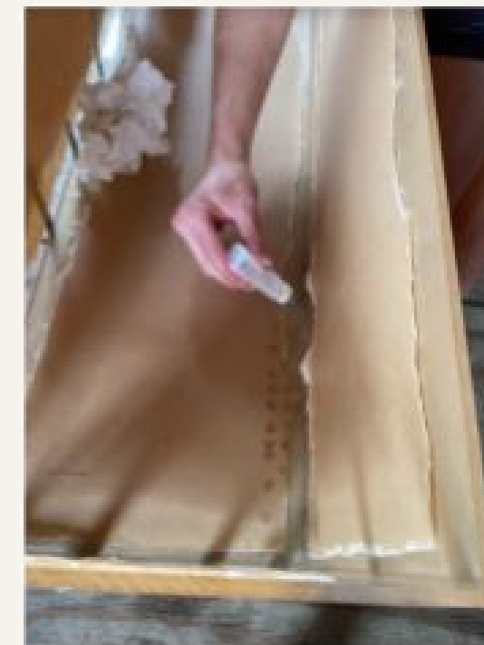
Applying acrylic cement
