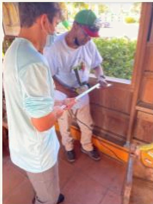
Creating metal frame for bottom of tank
