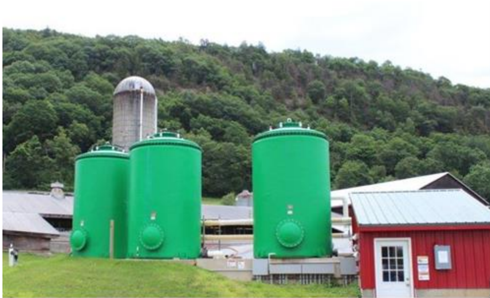
Figure 2.1: Barstow's Farm-Powered Anaerobic Digester. Reprinted from New England Farm Energy Collaborative (Barstows..., 2021, 'Blog Posts'). Copyright 2017 by Denise Barstow Manz. Reprinted with permission.
