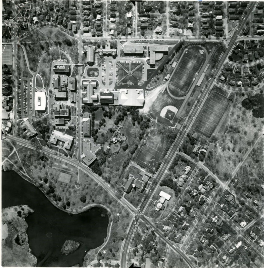
Figure 8. Aerial view of campus depicting West Street cutting through the middle, April 18th, 1968. Source: URL .
