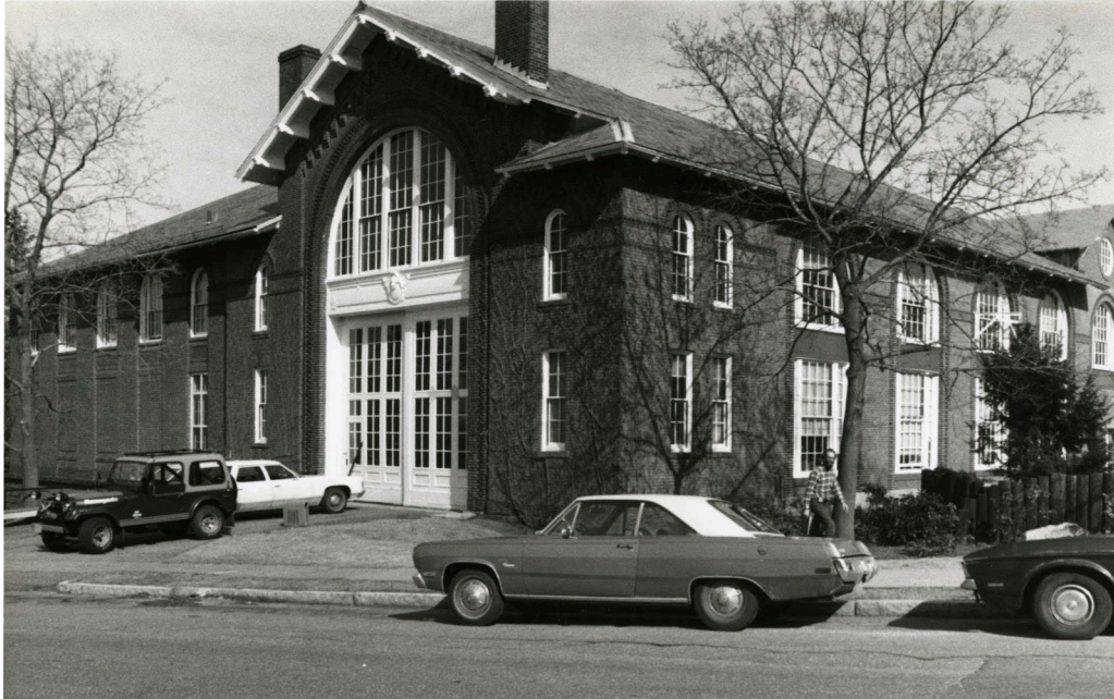
Figure 6. Exterior of Atwater Kent Labs, 1970-1979. Source: URL .
