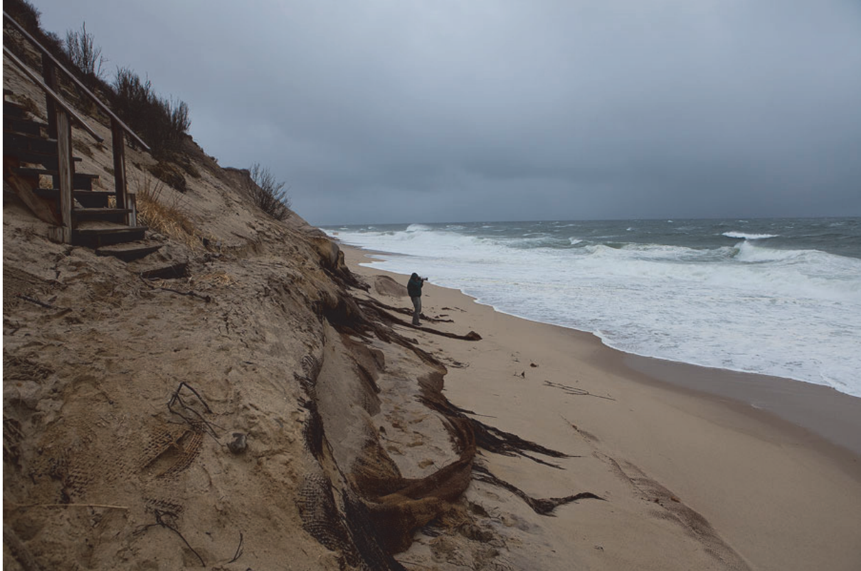
Figure 12: Photograph by Van Lieu Photography (2010): An Uncovered sandbag at the bottom on Siasconset Bluff
