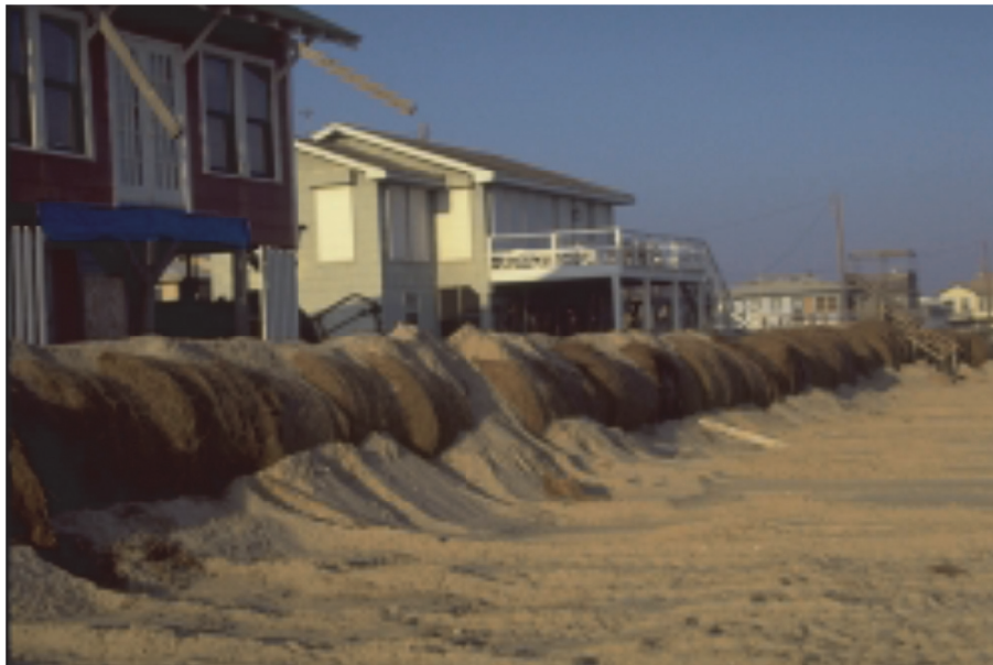
Figure 5: Use of hay bales as a protective barrier (Photo by Susanne C. Moser, February 1999)
