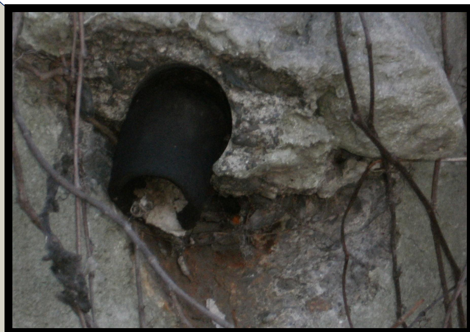
Drainage Pipe embedded in the side of the bridge © UWM Groups
