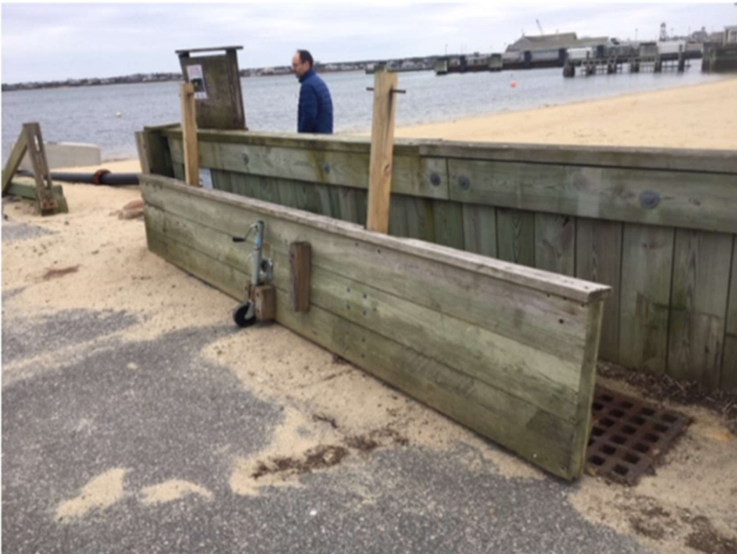
Figure 32: Children's Beach Tidal Gate (Fuss & O'Neil 2019)
