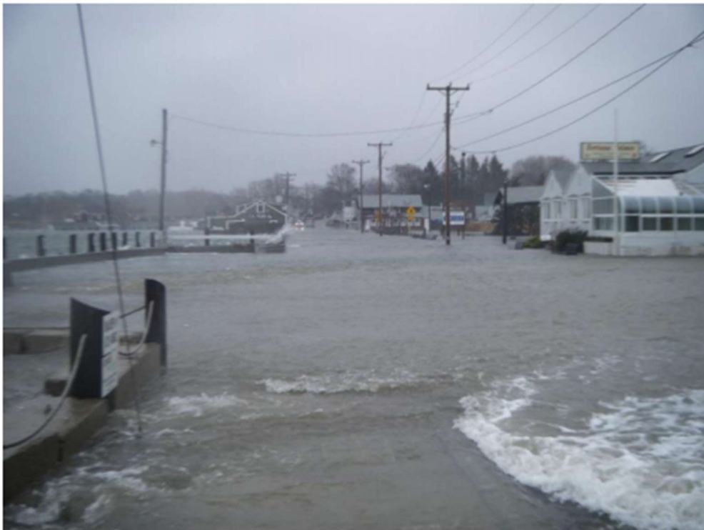
Figure 44: Image from the Essex HMP page 35 showing the "Essex Causeway" flooding. (Essex HMP, 2019, page 35)
