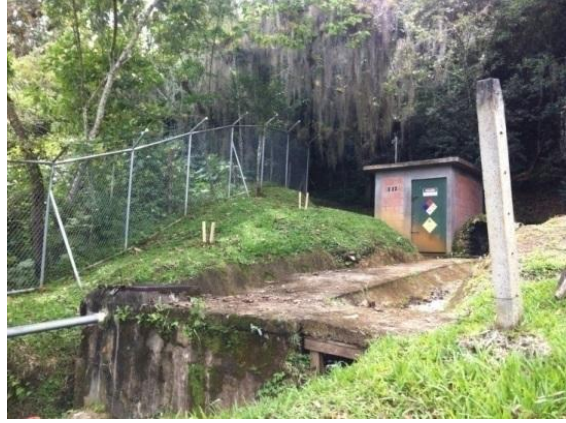
Figure 1: Ladrillera spring water supply system grounds
