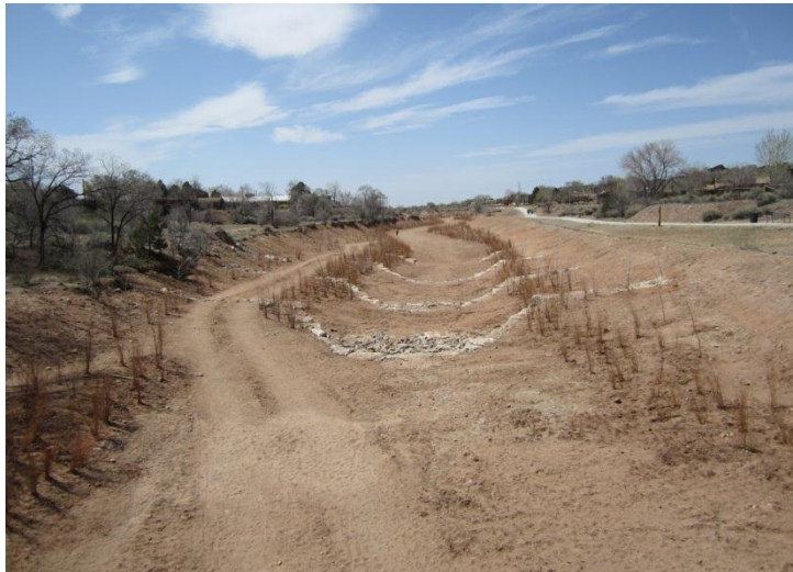
Figure 46: New River Construction at Frenchy's Field
