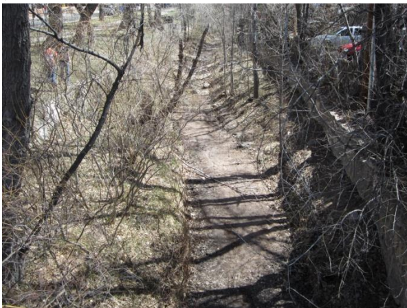
E Alameda & Paseo De Peralta – Upstream (3/28/12)
