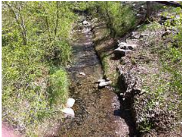
Brothers Lane Bridge – Upstream (4/10/2012)
