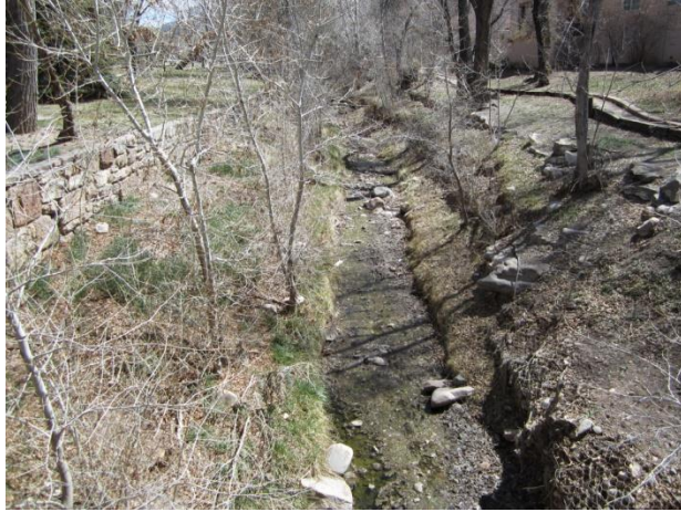
Brothers Lane Bridge – Upstream (3/28/12)
