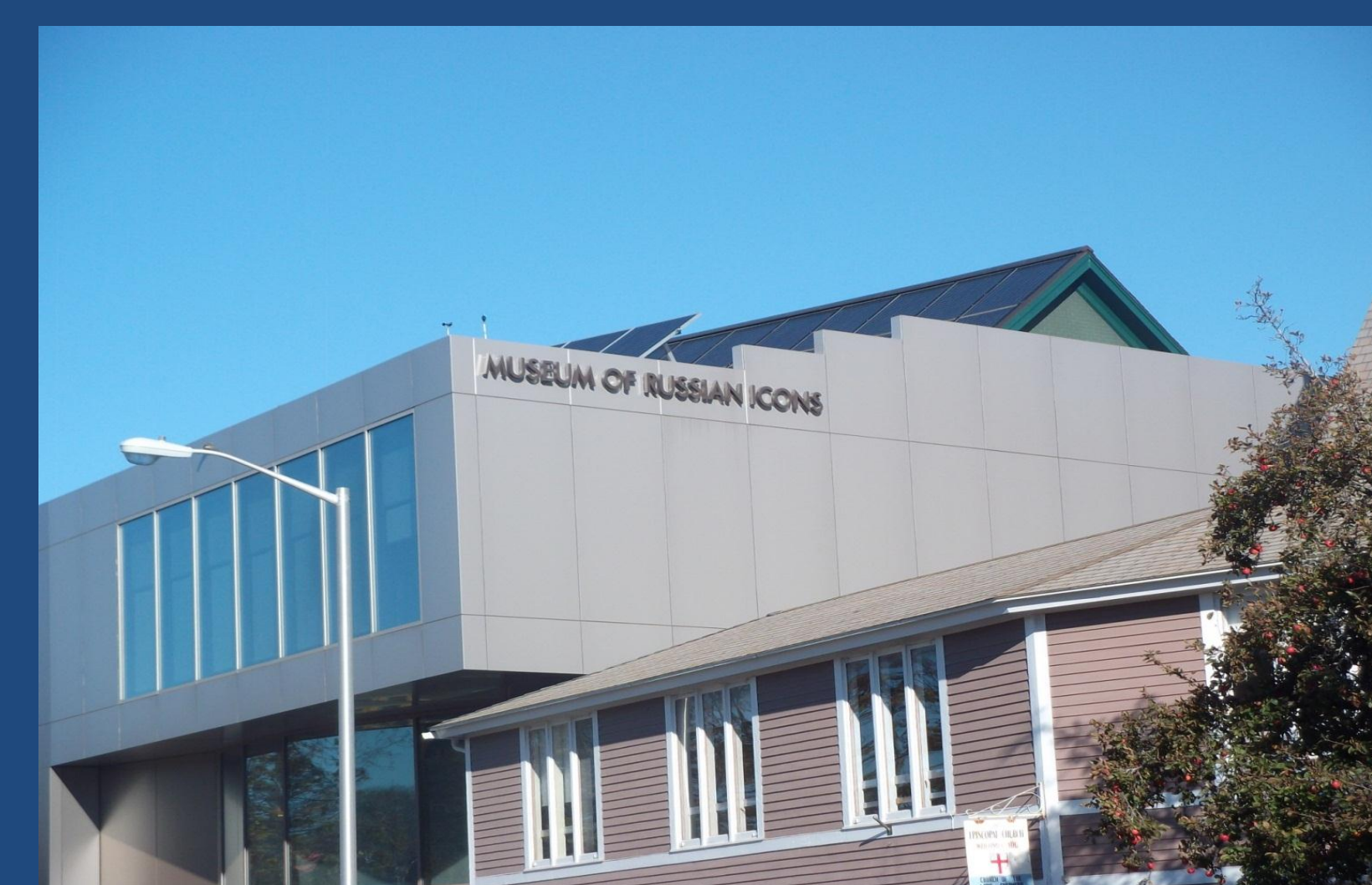
Back of the museum solar panels visible on roof
