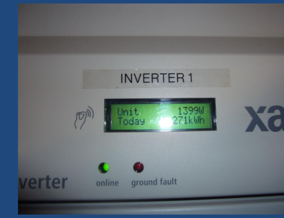
Inverter showing how much energy was produced by one module
