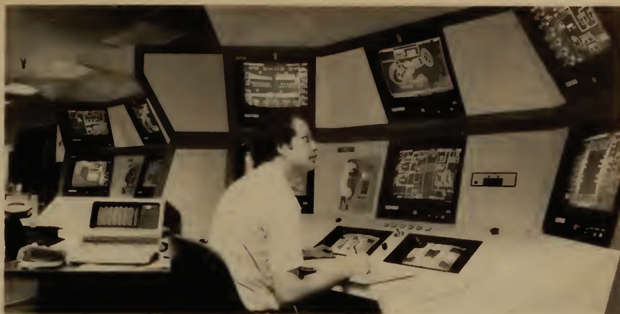
Bob Pancotti in control room
