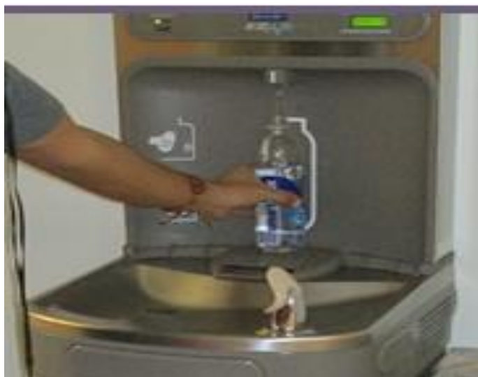
Figure 2.13: A water bottle refill station installed to help decrease plastic water bottle disposal
