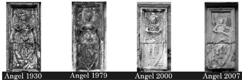
Figure 6: In 2007 a restoration attempt was made and the Angel was destroyed further
