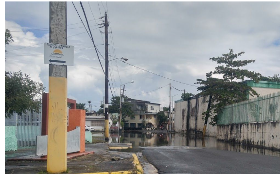
Figure 8: Flooded Street in Cantera
