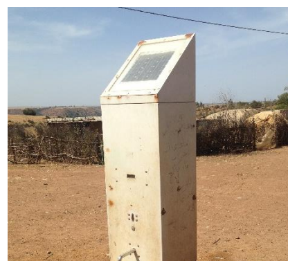
Figure 2: A solar powered, coin-operated water pump that pumps water from a well to provide drinking water for community members
