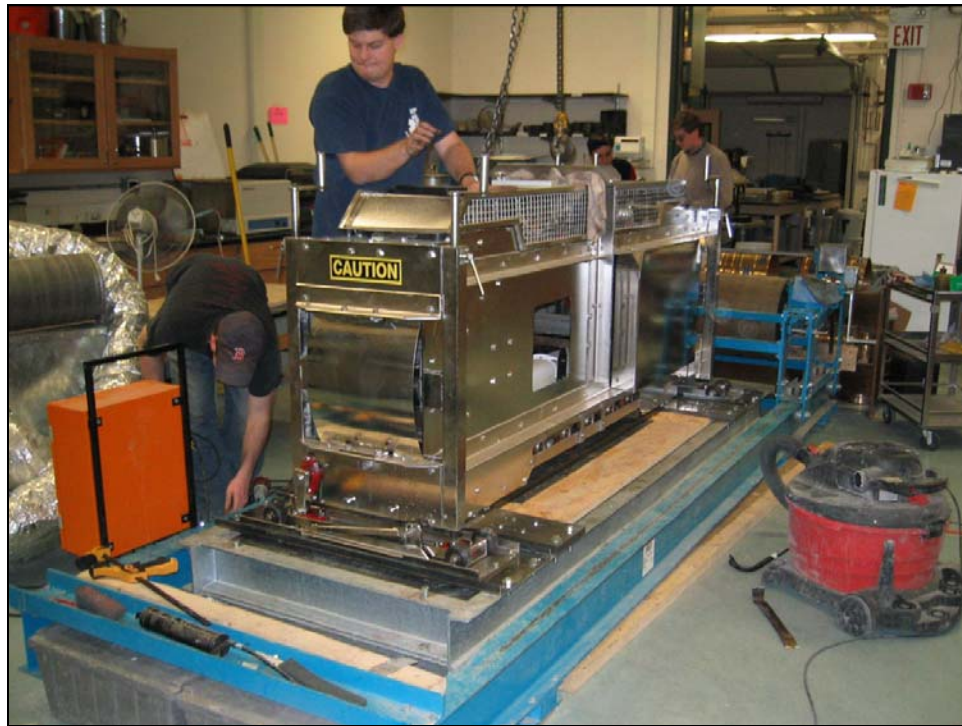
Figure 6.6 – Lowering MMLS3 into testing position and leveling (typical)
