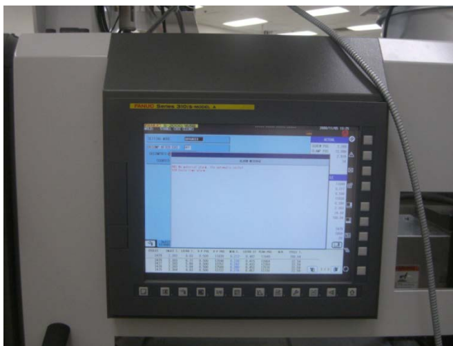
Figure 23: Molding Machine Central Control
