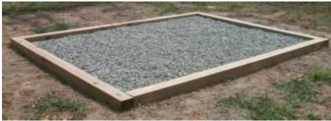
Figure 37 Crushed stone floor
