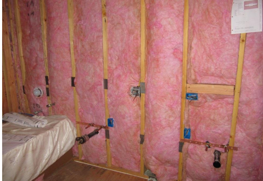
Figure 35. Double Skin Wall filled with Fiberglass
