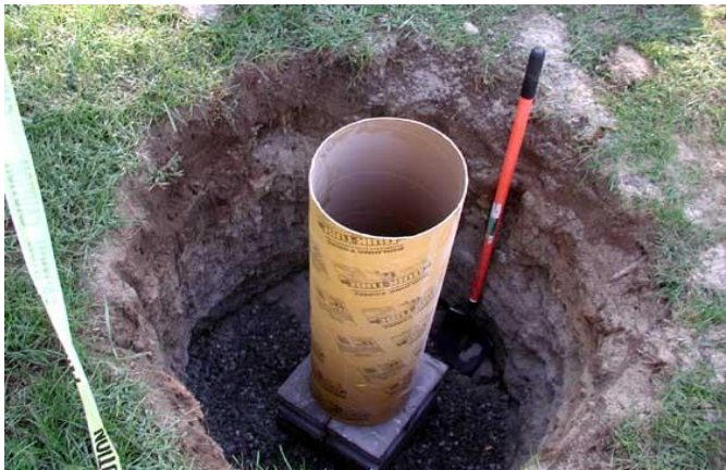
Figure 38. Sonotube being installed (Roberts J. , 2012)
