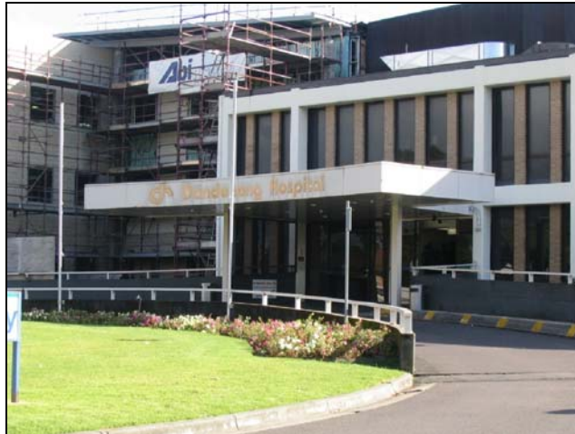
Figure 42: Front view of Dandenong Hospital
