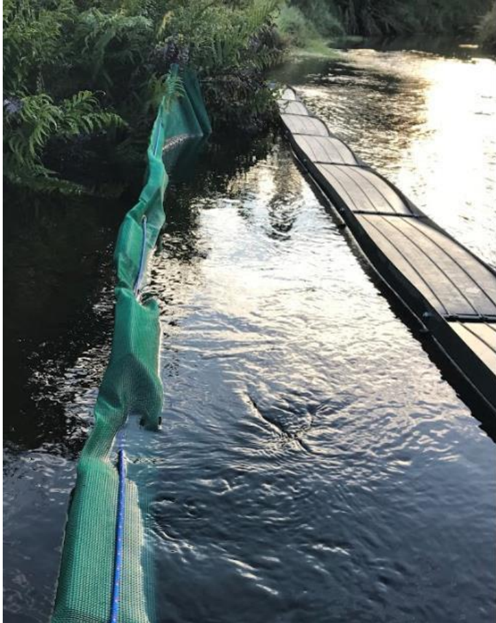
Figure 61: Mesh and boom system
