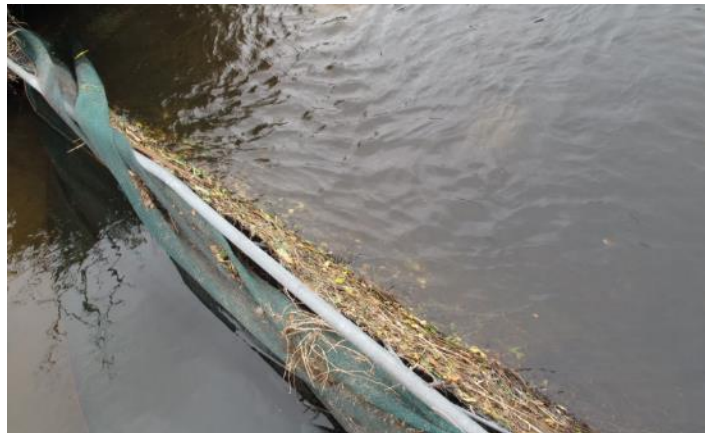
Figure 15: Close-up of previous intake debris solution (2016)
