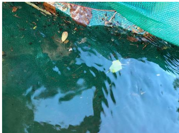
Figure 70: Debris on mesh
