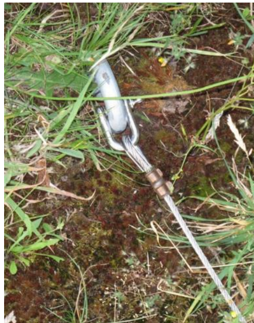
Figure 33: Floating wetland and anchoring system (2017)
