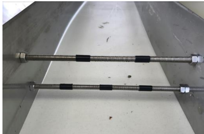
Figure 57: Electric tape around threaded rod to protect nylon
