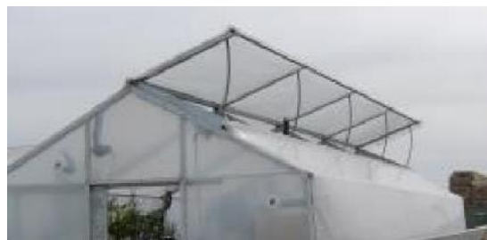
Figure 72: Ventilation design (Redpath)
