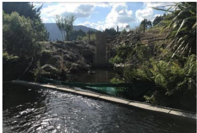
Figure 63: Full view of intake
