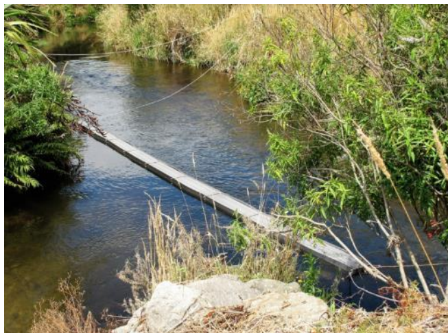
Figure 53: Boom's initial installation, anchored in front of the intake
