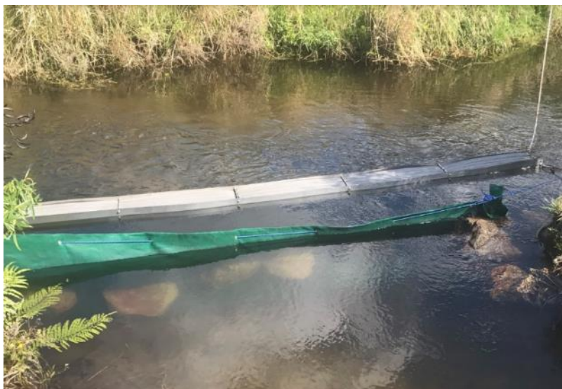
Figure 60: Mesh being held down by rocks
