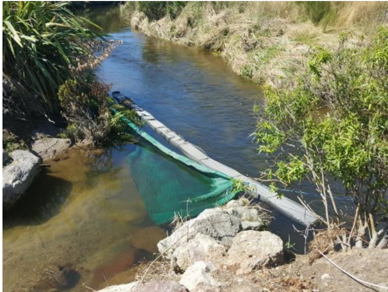
Figure 68: Boom back in the water after repairs
