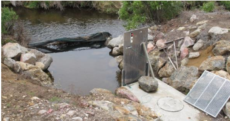
Figure 13: Intake with mesh gate (2016)
