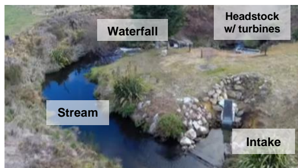
Figure 7: Aerial view of the stream and intake
