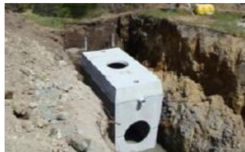
Figure 12: Septic tank intake (PowerSpout, 2014)
