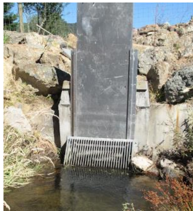
Figure 6: Micro-hydro Intake
