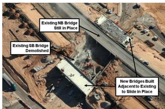
Figure 13: SIBC Construction Methods (UDOT/FHWA, 2013).
