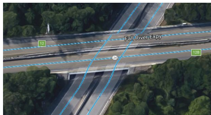
Figure 4: Aerial view of Rte. 24 bridge (Google Maps).
