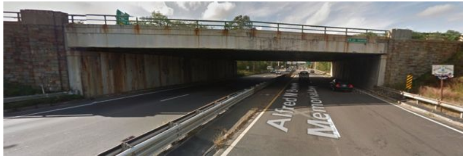
Figure 5: Route 24/140 Interchange (Google Maps).
