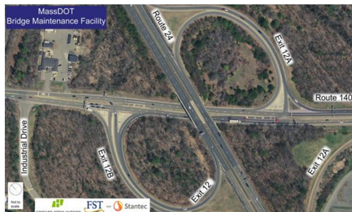
Figure 1: Route 140/Route 24 Interchange Existing Conditions.
