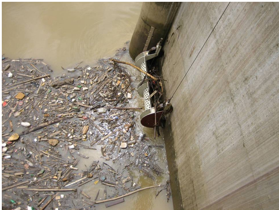
Figure 19: Clam Used for Debris Removal
