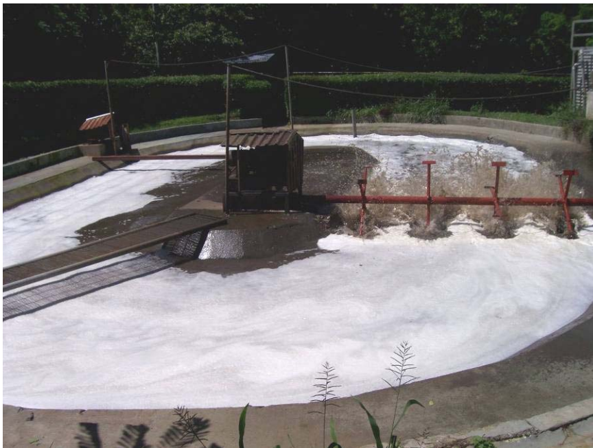
Figure 31: On-Site Wastewater Treatment Facility
